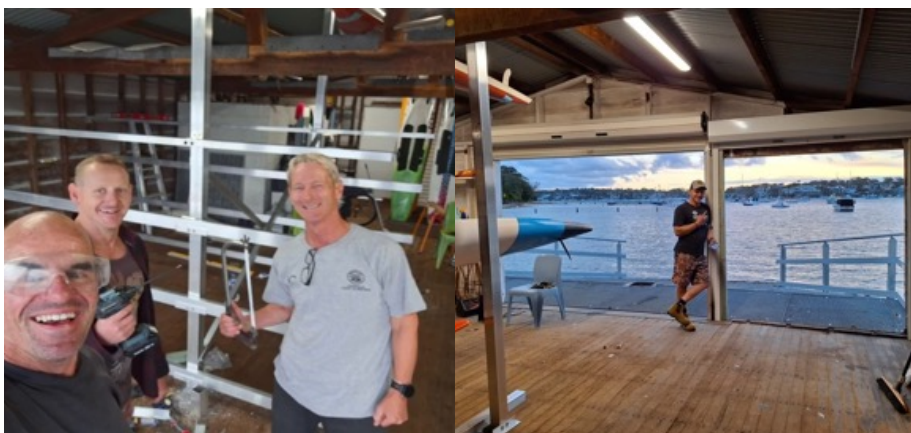
Chris Freeman, Chris Chambers and Greg Cooper kept themselves occupied while the team was battling the surf at Maroochydoore replacing the ski racking and installing a new roller door at the Gunnamatta Bay shed. This will make it a safer environment and enable our younger members to train on accessible craft – boats, skis, boards and nipper equipment.
