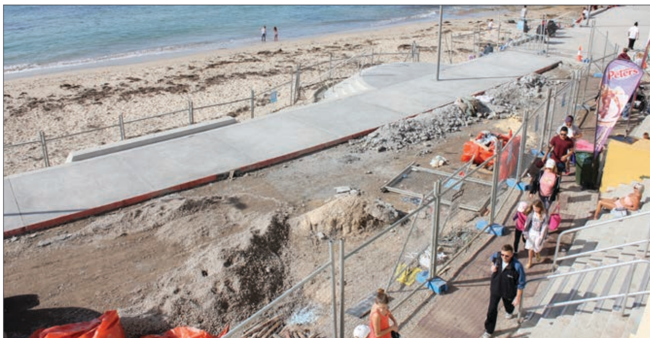
Promenade works July 2013
