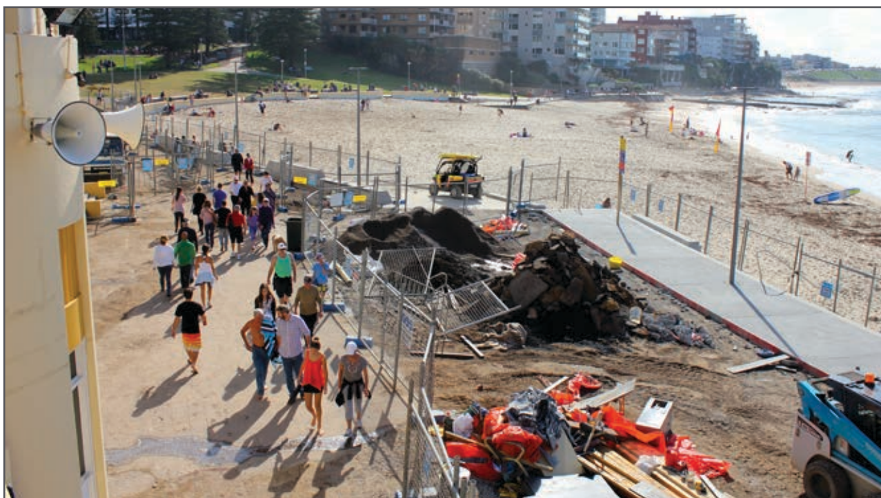
Promenade works July 2013
